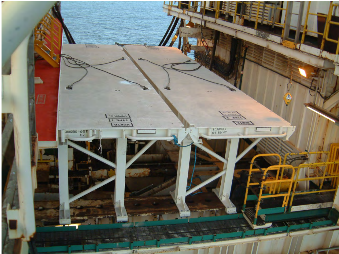
(ANDREW - CRI DROPPED OBJECTS PROTECTION - SECTIONS 1, 2 & CANOPY - IN LOCATION)
