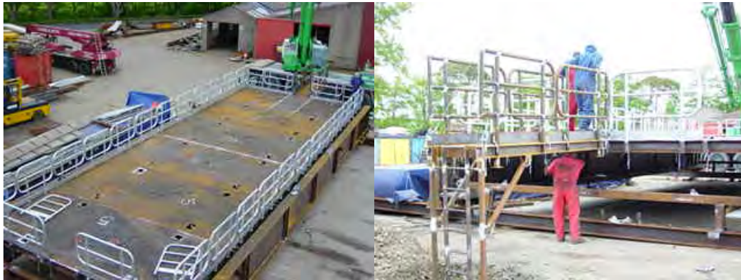
(NORTH ALWYN - LAYDOWN PLATFORM TRIAL ASSEMBLY)
