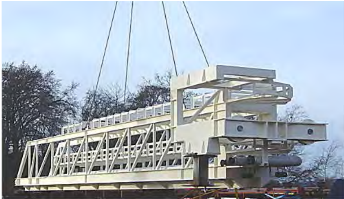
(MAGNUS - EAST/WEST DRAG CHAIN REPLACEMENT STEELWORK)
